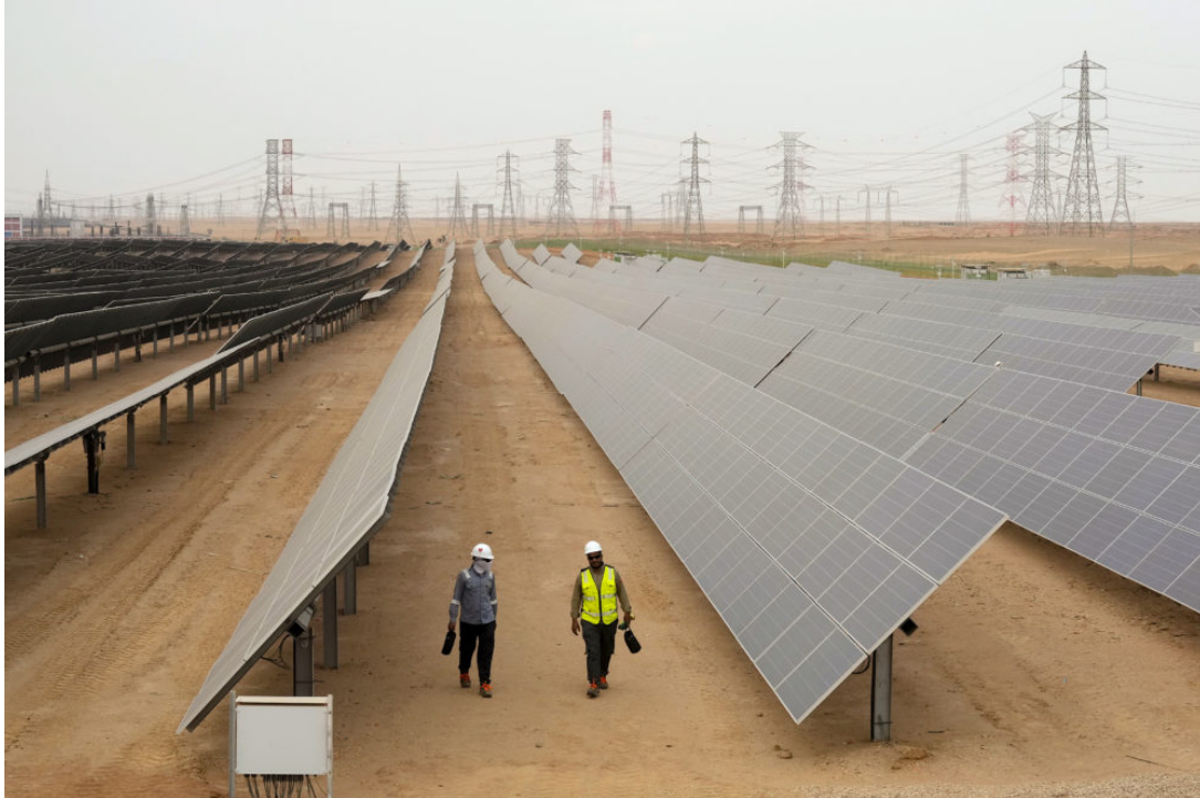
The Benban Solar Park in Aswan, Egypt. AMR NABIL / AP PHOTO
