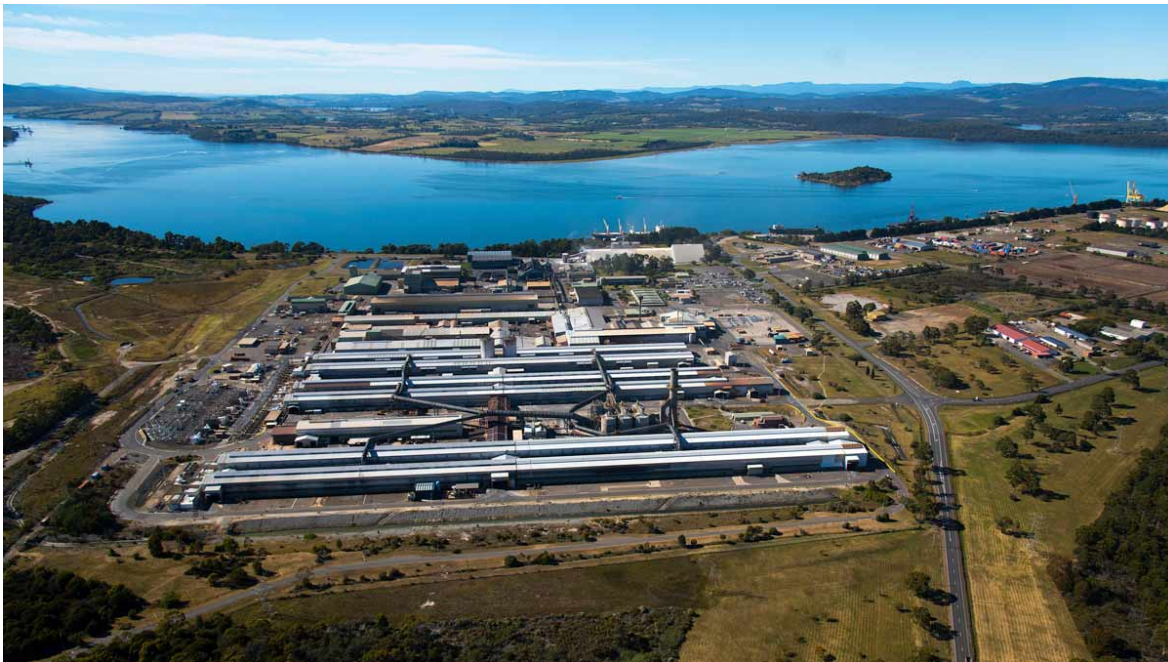
The Bell Bay aluminium smelter (Photo credit: Rio Tinto).
