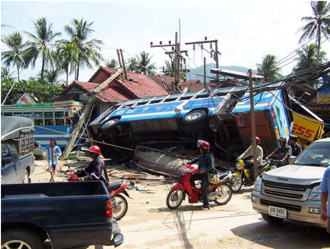
Buses and boats blocked streets. Note the 220 Volt electrical line with temporary pole (photo Dec. 27)
