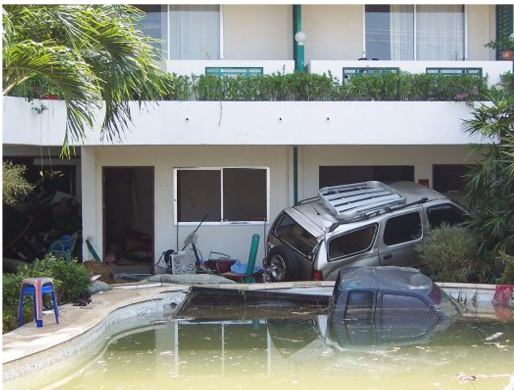
Car and debris filled the room on left (photo Dec. 27)
