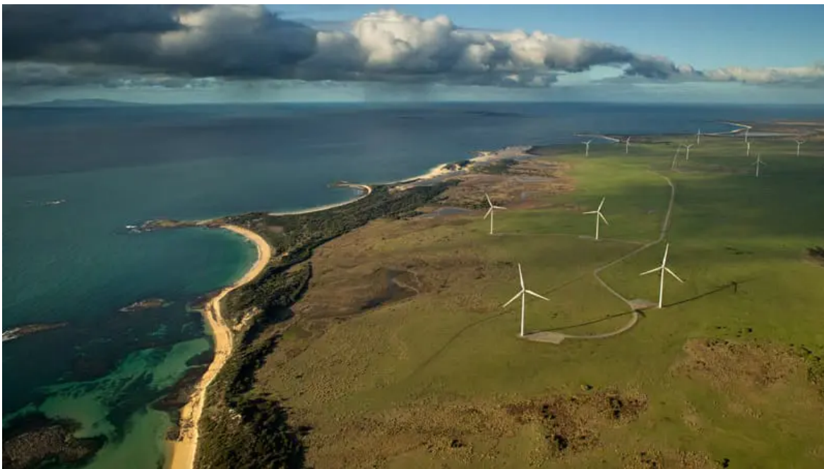
Musselroe Wind farm in Tasmania
